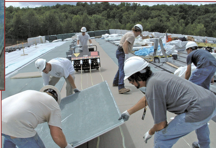
Figure 3 – Two-part polyurethane adhesives are low VOC options for installing board stock or fleece-back membranes.
