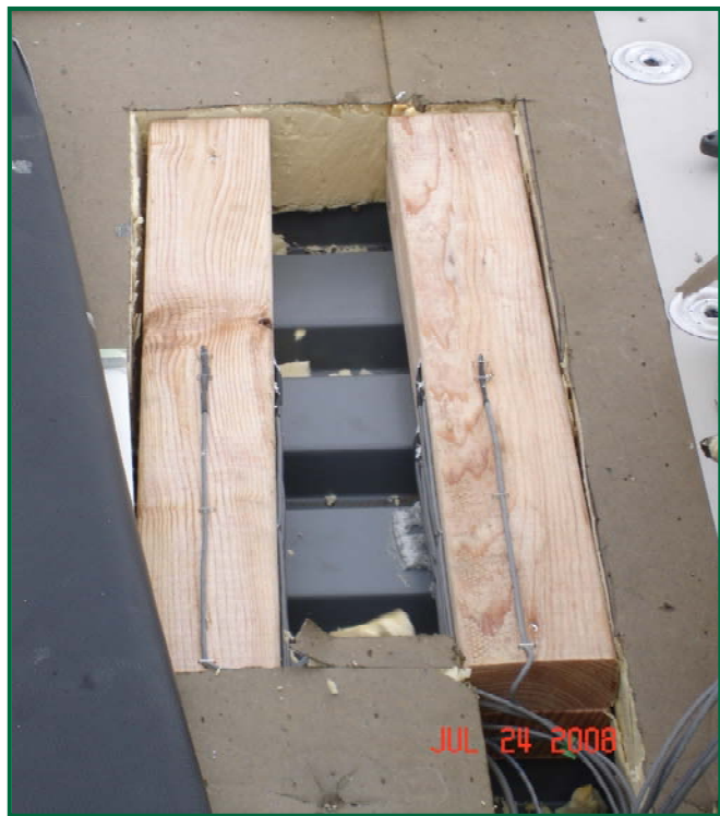
Figure 13 – Simulated wood nailers installed on roof deck
