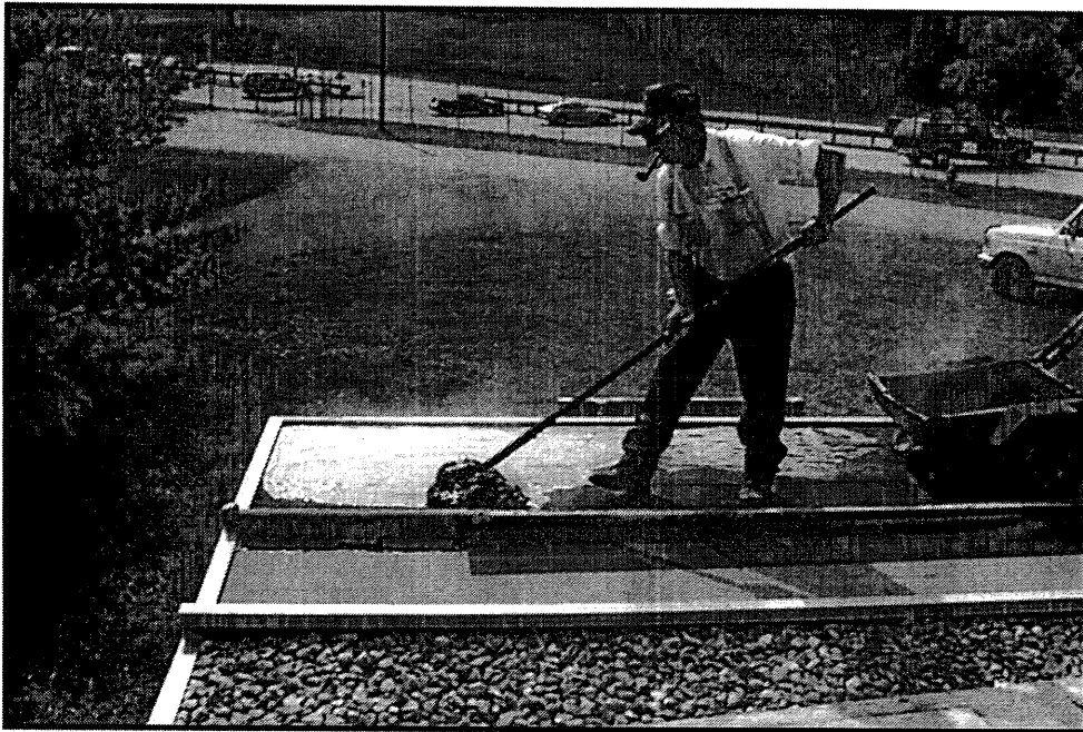
Fig. 5. The BUR is made of four alternating layers of bitumen and bitumen-saturated felt paper.
